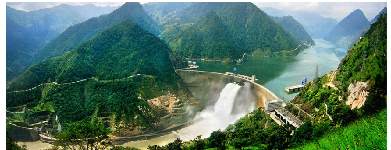
The Bank provided support for Yalong River green power project
