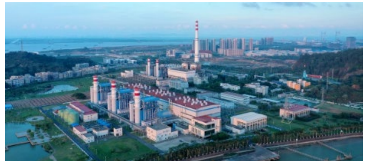
The Bank facilitates power companies to accelerate technological upgrading for energy conservation
